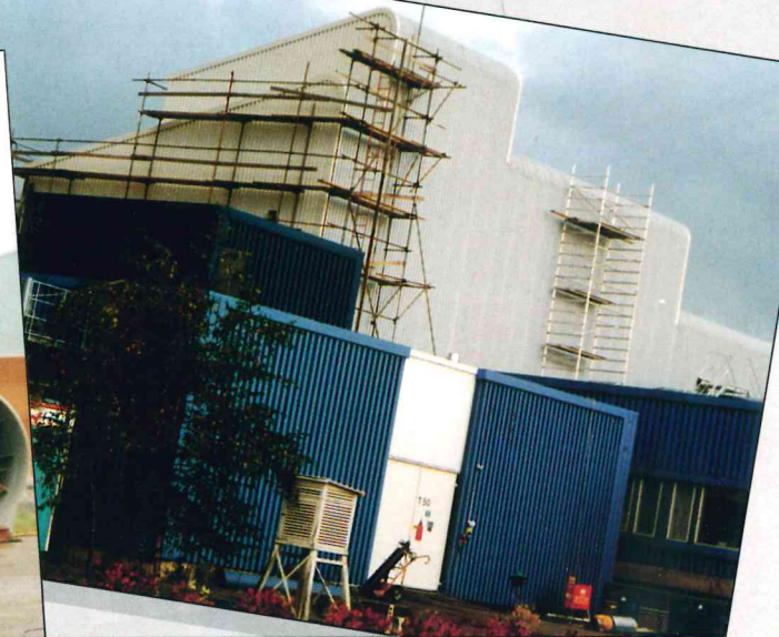
Klimatvindtunnel, Volvo Göteborg
